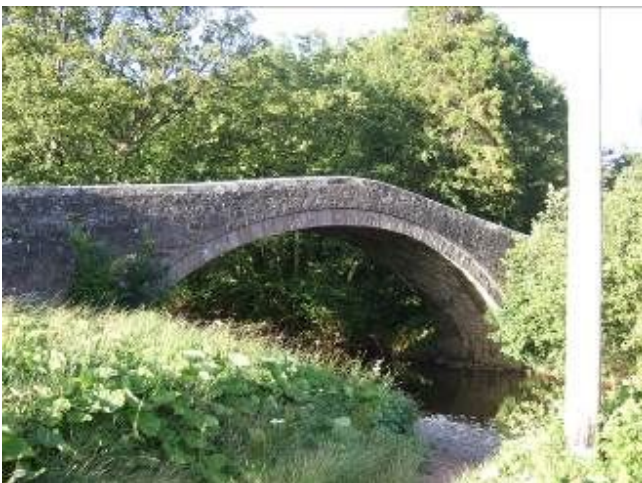
BELL BRIDGE IN 2010.
