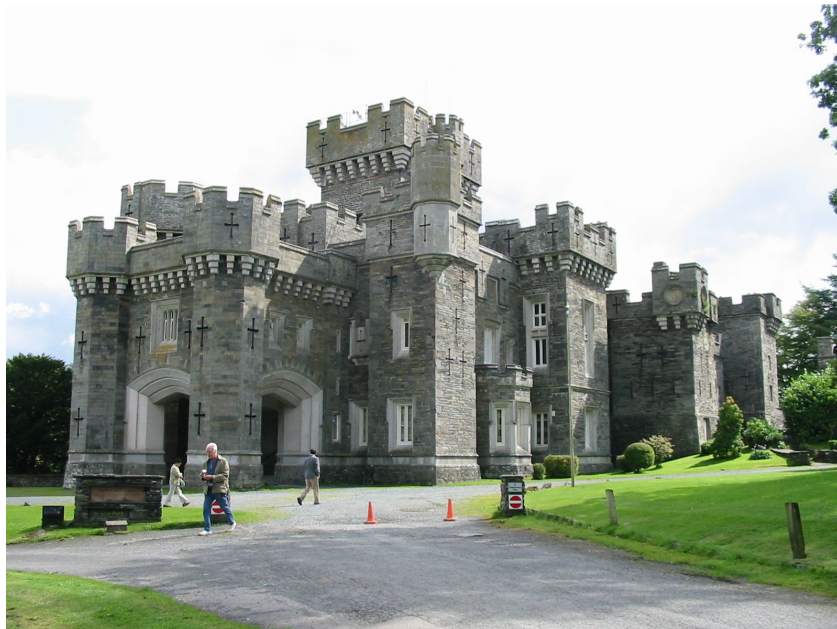
Wray Castle near Hawkshead. Water was supplied from tanks on the roof and warm air from stove rooms under the terrace. Photo Roger Baker.
